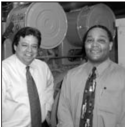
Mark Gonzales, director of hospital construction projects, and Herschel Johnson, associated director of DCM, in front of one of the new emergency generators.
