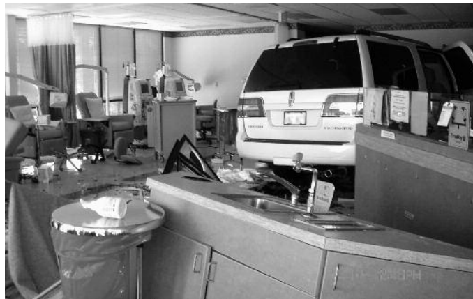
When a vehicle traveling Rainbow Boulevard crashed through the Dialysis Center Saturday, May 17, dozens of dedicated hospital staff members pitched in to help transfer dialysis services to Unit 45.
